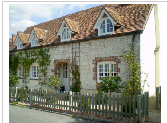
Chalk block cottage with brick framing. Manor Cottage, Blewbury.
