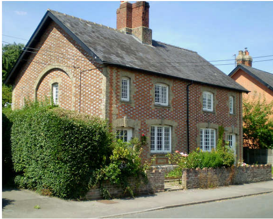
Combined red and grey patterned brickwork. Great Bedwyn. This brick pattern known as Flemish bond was very popular in the 19 th Century. The unglazed red bricks are laid horizontally (stretchers) and the grey bricks are laid end on (headers).
