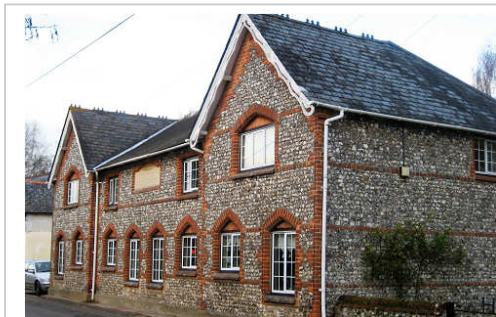
Flint and brick house, St Mary Bourne
