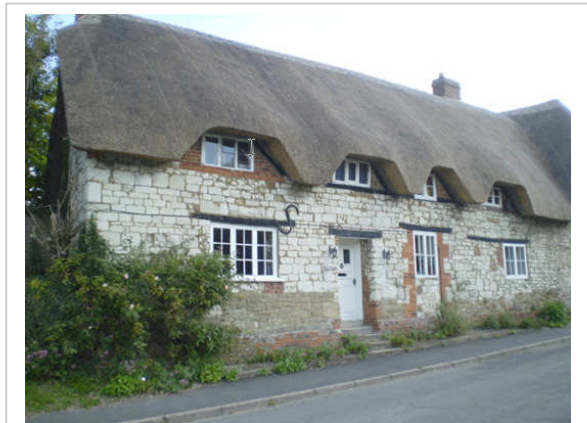
Chalk block cottage with brick and sarsen foundations and wooden lintels. Ashbury.
