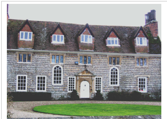
Alternating courses of cut sarsen and flints. Manor farm at Odbourne Maizey.
