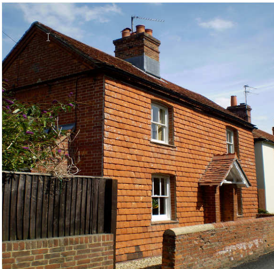
Tile-hung gable end. Butts Cottage, Kintbury.
