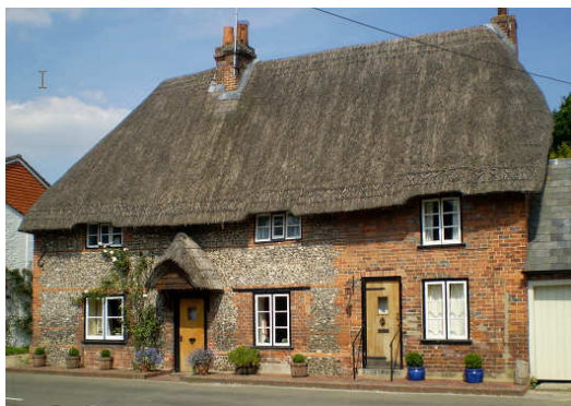
The Old School House, Hurstbourne Tarrant with thatched roof, rough flint walls and brick framing.
