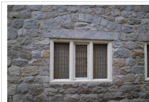
Cut sarsens laid in courses, Avebury Manor Stable
