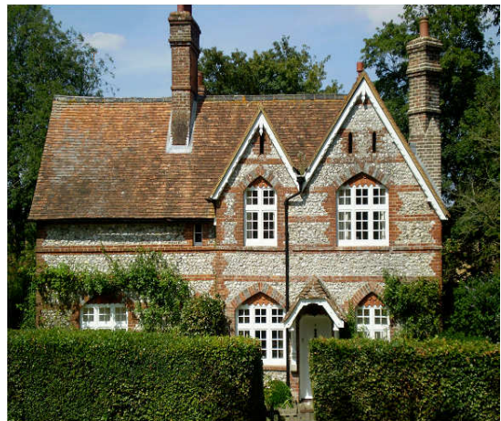
By the 19 th century, brick and flint were being used in combination for decorative effect. Mid-19 th century use of flint with interspersed brick courses and brick framing. Oxenwood.
