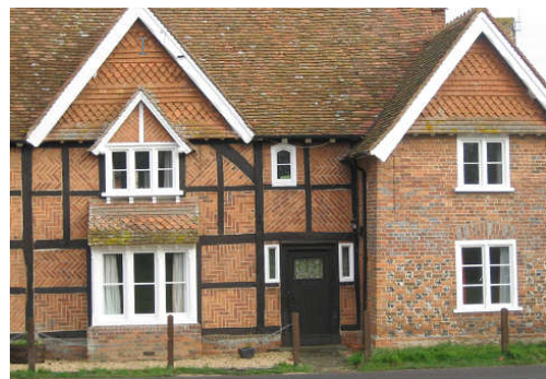
Timber-framed house with elaborate chevron-patterned brick infill and tile hunchable. Chilton House, Chilton.
