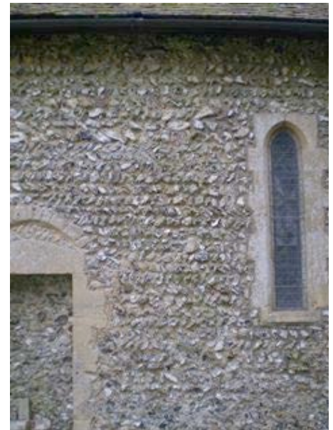
Swyncombe church: field flints in roughly-coursed rubble walls.
