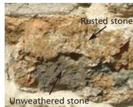
The ironstone is vulnerable to weathering. The acid in rainwater reacts with the calcite minerals in the ironstone and dissolves them away. This causes the building stones to crumble and flake. Look out for examples of this in the village.
